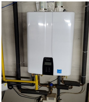
Figure 2.2 South Yard Tankless Water Heater
