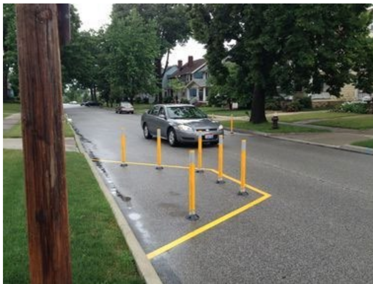
Temporary chicane installation
