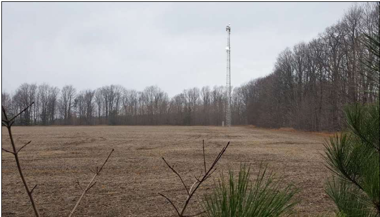
Photo Rendering of the Proposed 45m Lite-Duty Self-Support Lattice Tower Co-Location Opportunities Considered:
