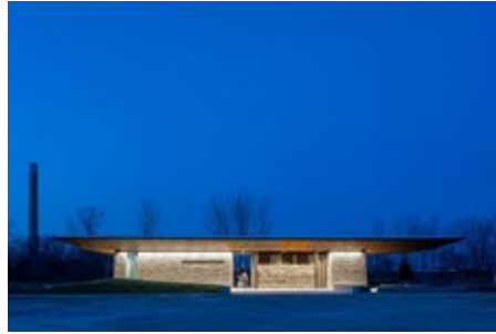
Tommy Thompson Park Entrance Pavilion, Toronto, Ontario
