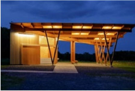
Tommy Thompson Park Entrance Pavilion, Toronto, Ontario
