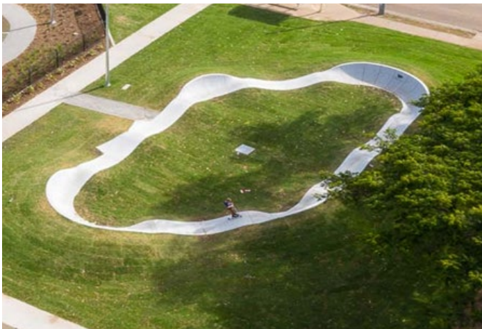
Paved Pump Track
