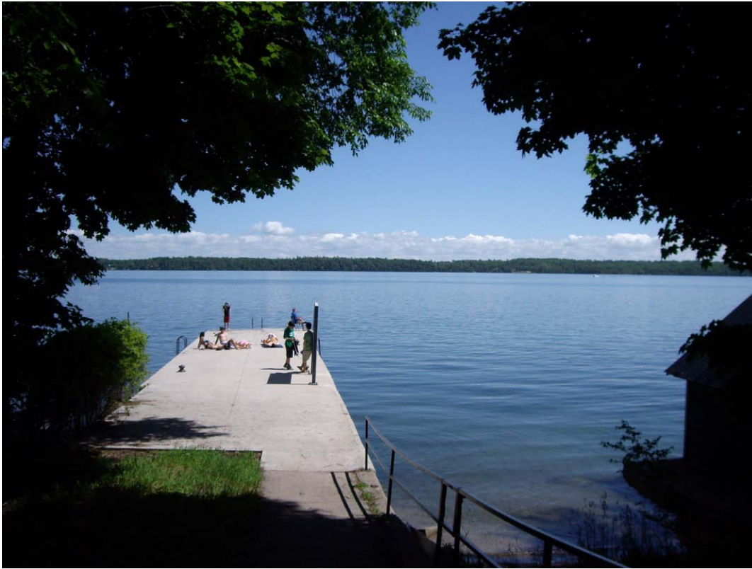
Figure 52: Shanty Bay Wharf
